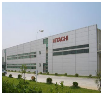
Hitachi Construction (Suzhou 14 units)
