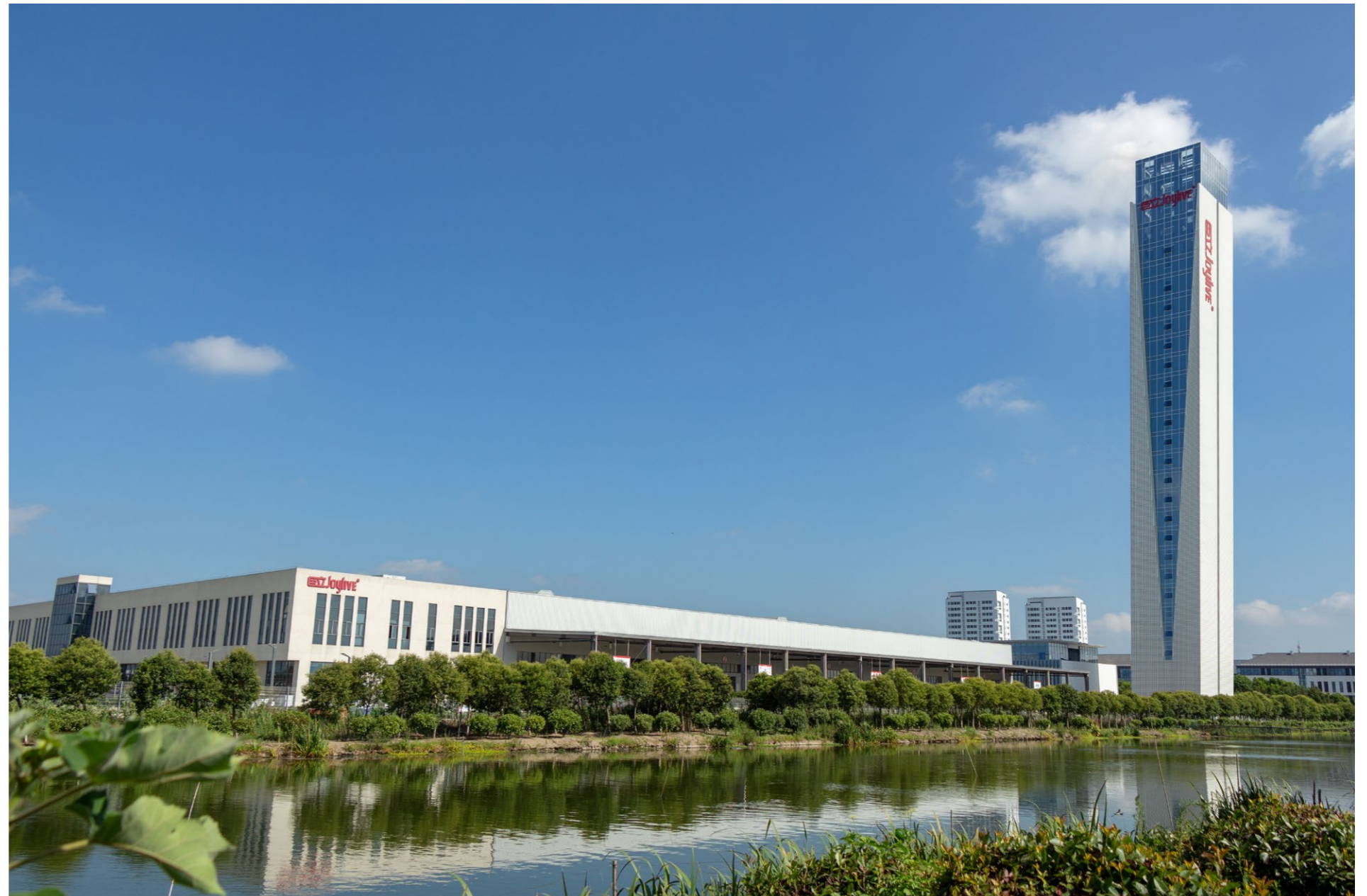
70, 000 m2 area manufacturing factory with 118 m height test tower
